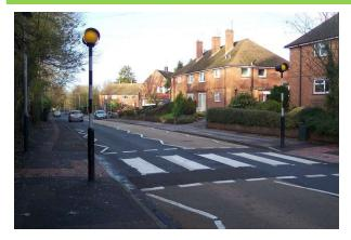
Where pedestrians are having difficulty crossing a road, a new zebra crossing may be a suitable solution to deal with this issue. They consist of dropped kerbs, tactile paving, belisha beacons on posts and sometimes high friction surfacing on the approaches to help vehicles stop quickly.
