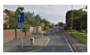
It is worth noting that there are unfavourable side effects to most types of calming. Speed humps and cushions for example can cause unwanted vibration and noise for nearby residents. Chicanes and narrowing may result in the loss of on-street parking and can increase noise levels, cause congestion and, in extreme cases, lead to road rage incidents.
