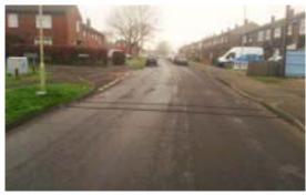
ATC tube survey which consists of a pair of tubes laid across the carriageway which are connected to a data logger that allows reports such as traffic volume, speed and vehicle classification to be generated. This type of count would generally be carried over a 7-day period.
